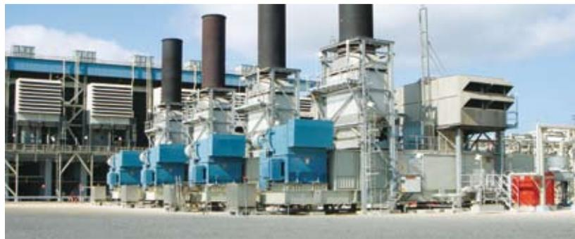
Four SGT-500 units installed in Egypt to power an LNG plant.
